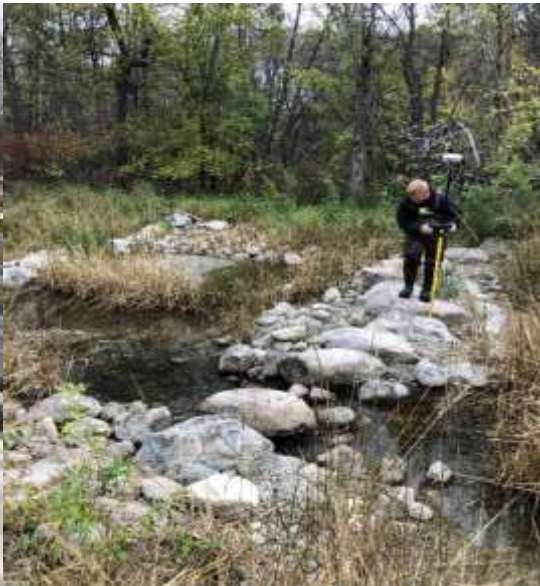
Surveying Fish Passage Elevation.
