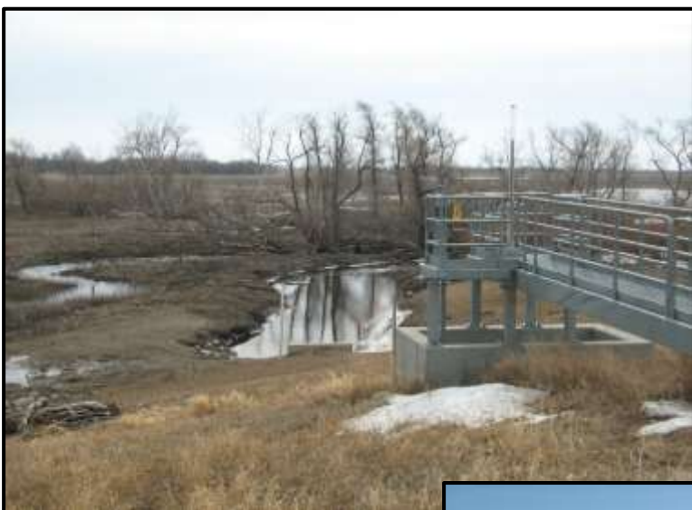
Example of a “Dry” Impoundment. Stored flood water is released as soon as downstream channel conditions are acceptable to pass flows.
