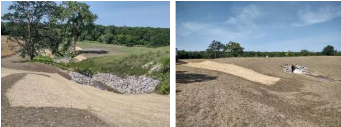
Outlet to Red Lake County Ditch 62
