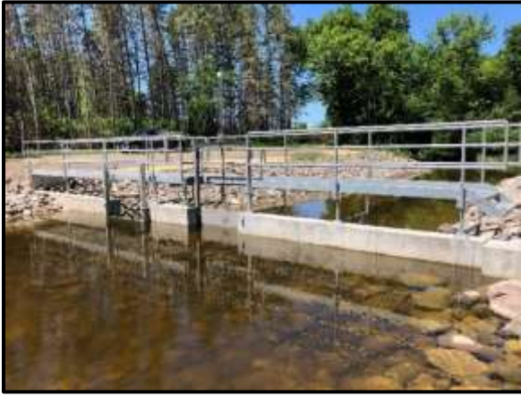
New structure with gates and catwalk.
