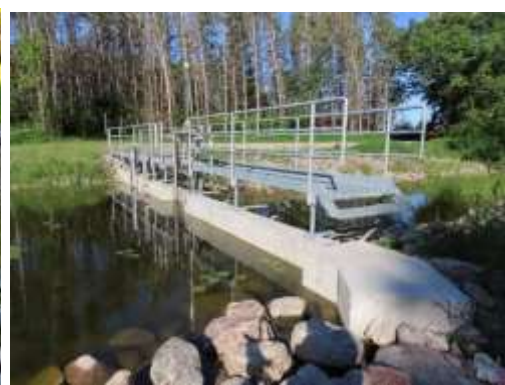
Outlet structure without steel gates and catwalk
